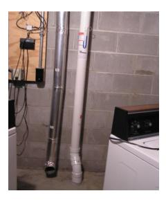
In this picture, a PVC pipe is connected to an existing drain tile under the foundation of a home. The performance indicator (blue tube) shows the fan is working.
