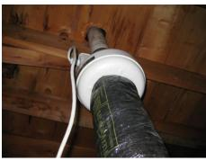
The radon fan should be located in an unconditioned space, such as the attic or outside. This fan will pull the radon gas from the soil and help expel the gas above the roof line.
